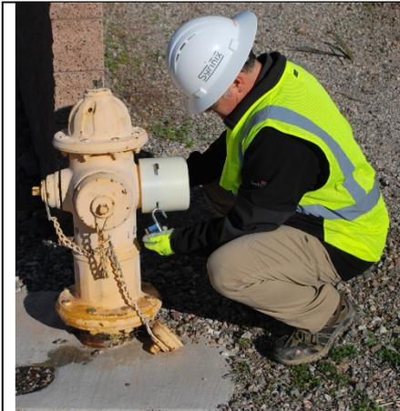
STEP 8: Secure with the locking-bars and padlock.
